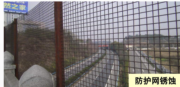
防护网锈蚀、破损
