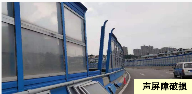
防护网锈蚀、破损
